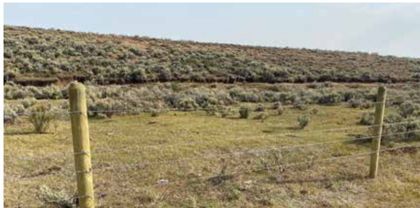
A bottom barbless wire at least 18" from the ground aids passage for pronghorn and other wildlife. Credit: WGFD.
