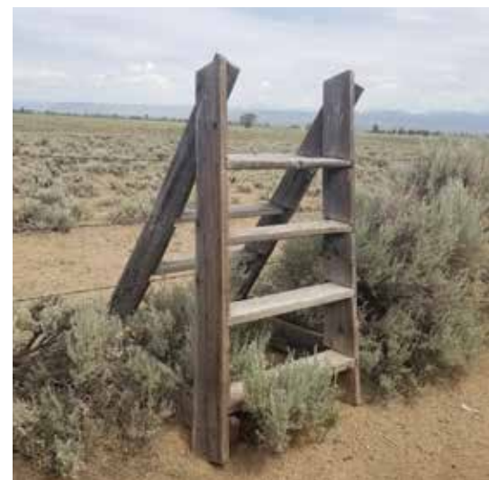
A V-gate (left) or fence ladder (right) allows humans on foot to cross easily without the risk a gate will be left open inadvertently. Photo credits: (left): Christine Paige, (right) WGFD.
