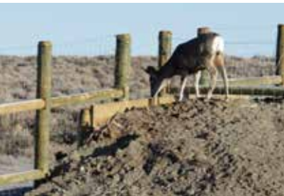
A 7'-8' fence is an effective barrier to elk and deer, but should be used only for specific needs such as gardens, haystack yards, or as highway wildlife barriers in conjunction with wildlife crossings and jump-outs. Credit: Mark Gocke, WGFD.
