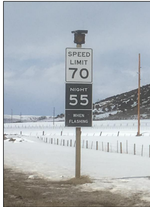
Figure 2. Photo. Split daytime and nighttime speed limit sign with flashing beacon.
